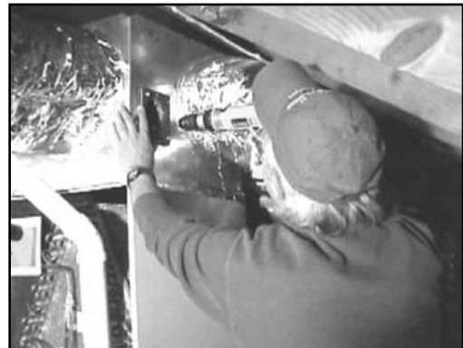
2. Install mounting plate over the opening. GL136 can be mounted in any rotational direction, as long as safety switch pin is aligned with hole in unit (2 o'clock shown here).
