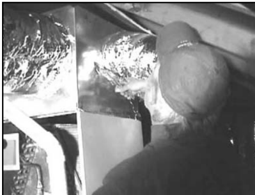
1. Use mounting plate to check for clearance. Mark plate hole, then cut a 3½” hole into the plenum downstream of the A/C coils.
