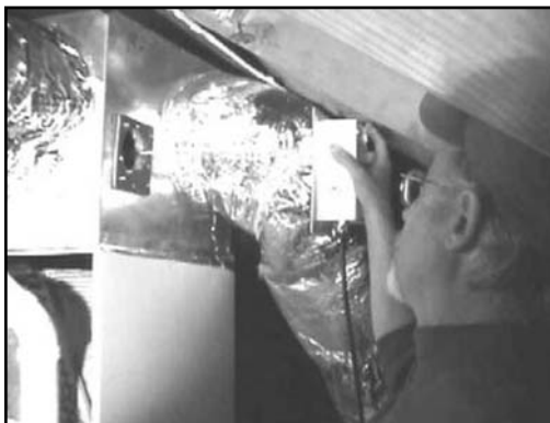
3. Install lamp into device, then insert device (with lamp through hole) onto mounting plate. Note: If installing GPCO grid, insert GPCO through mounting plate before lamp and unit.
