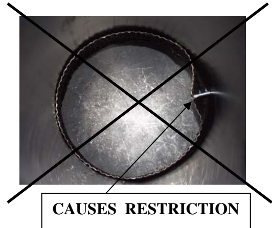
FAULTY INSTALLATION
